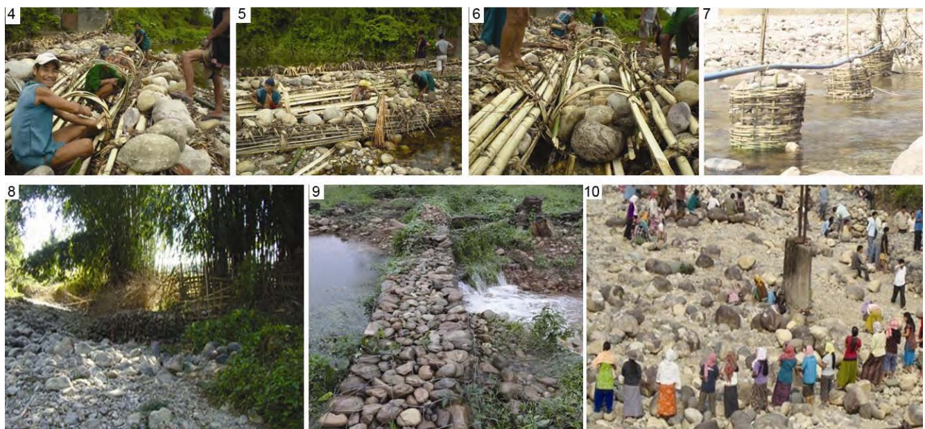
Fig. (4-10) – Fig. 4—Panikheti based on Yetbung Lingang structure; Fig. 5—Schematic diagram of Yetbung Lingang ; Fig. 6—Filling of stones in the frame Yetbung Lingang ; Fig. 7— Linkum as a support for laying pipeline across the small river/stream; Fig. 8—Stream bank erosion is prevented by Linkum ; Fig. 9— Linkum as filtered check dam prevents gully erosion; Fig. 10—Community making Gabion-Linkum structure for protecting the stream banks
