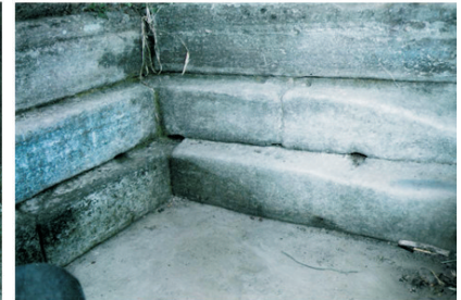
Fig.6 Internal view of Naula
